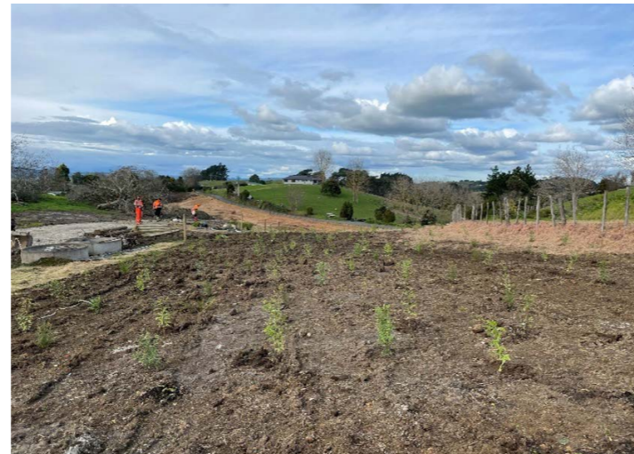
New planting underway in ridge section.
