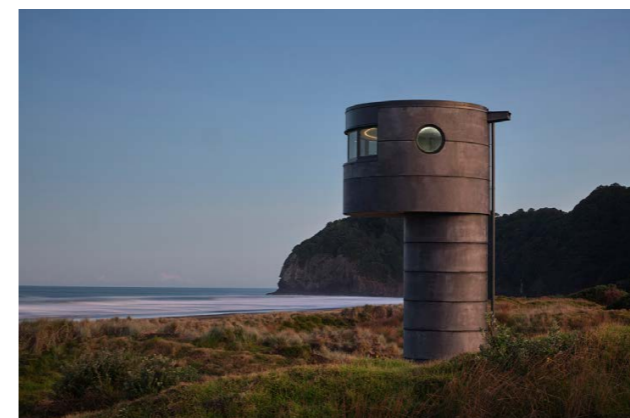
As well as greatly improving the safety and patrol capabilities, the structure is also designed to fit perfectly with its surroundings
